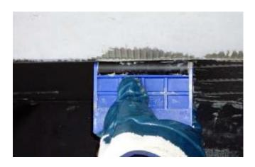
2. Apply the Pro-Elast with a roller making sure no air bubbles remain under the foil. Overlap ends at least 4" and use Inno-Elast® glue to seal all edges.
