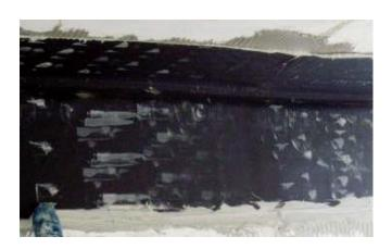
3. Allow Pro-Elast curing time as outlined in Technical Data Sheet, making sure to protect Pro-Elast® from any external damage while curing.
